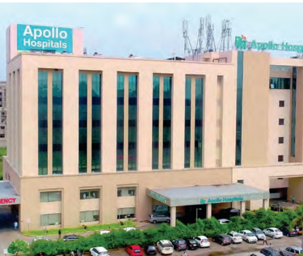
BELOW Apollo Hospital, Visakhapatnam, is an MEP project executed by Blue Star
