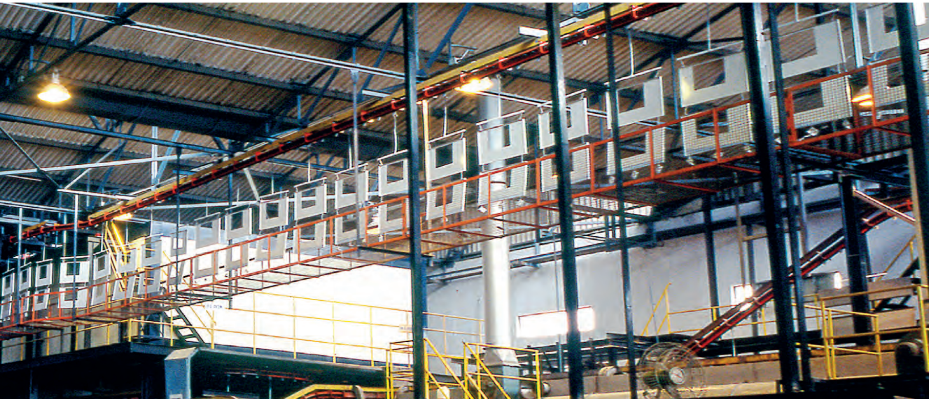
Paint shop at Dadra Plant
